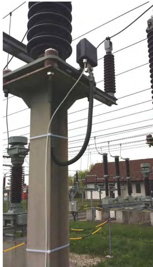
The data cable is weather- and UV-resistant and made for outdoor installation. We do not recommend to lead the cable through pipes or canals to prevent cable damages and influences to the data transmission.
